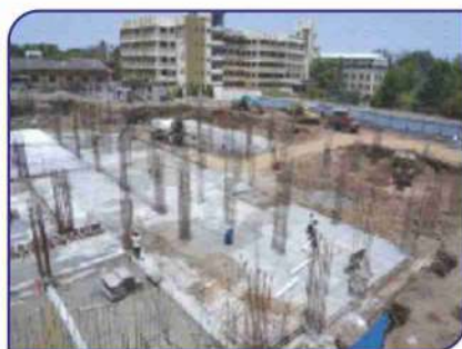
Hospital Work in Progress
